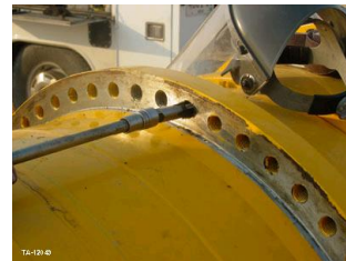
Cleaning paint and rust prior to torquing
